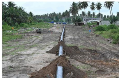
New route: Pipelines under construction to transport natural gas from platforms off the coast of Jacqueville in Ivory Coast. FILE PHOTO
