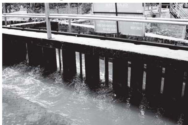
Fig. 18.4 Grit and sand removal tank
