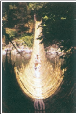
Figure 6.7 : Rope Bridge (Arunachal Pradesh)
