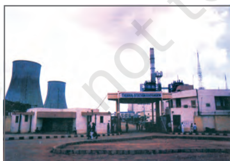
Fig 3.10: A view of a Thermal Power Station
