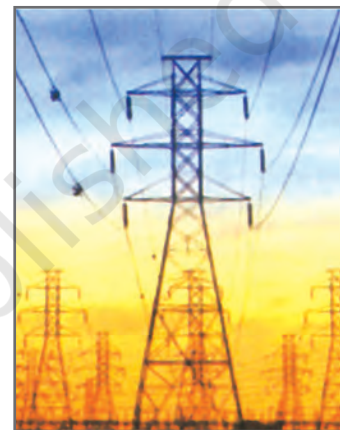
Fig. 3.7: National Power Grid to supply Electricity
