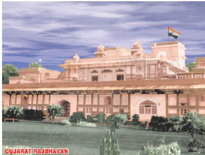
Figure 19.1 Raj Bhavan, Ahmedabad
